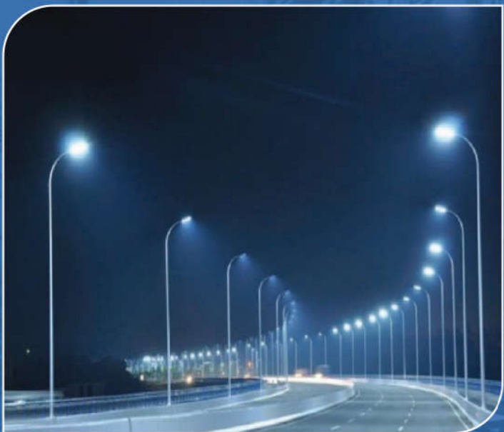
Traffic lighting system
