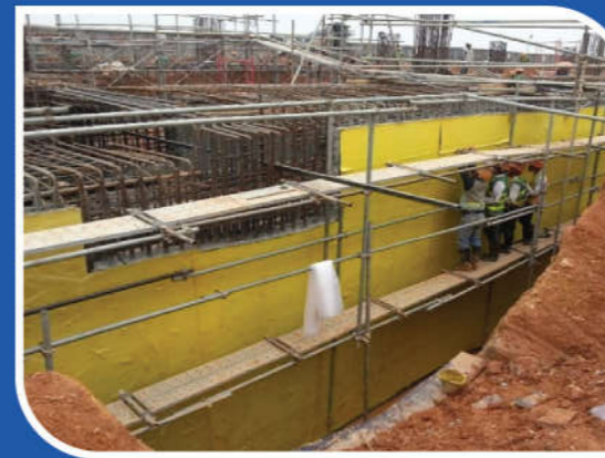
Waterproof layer for tunnel
